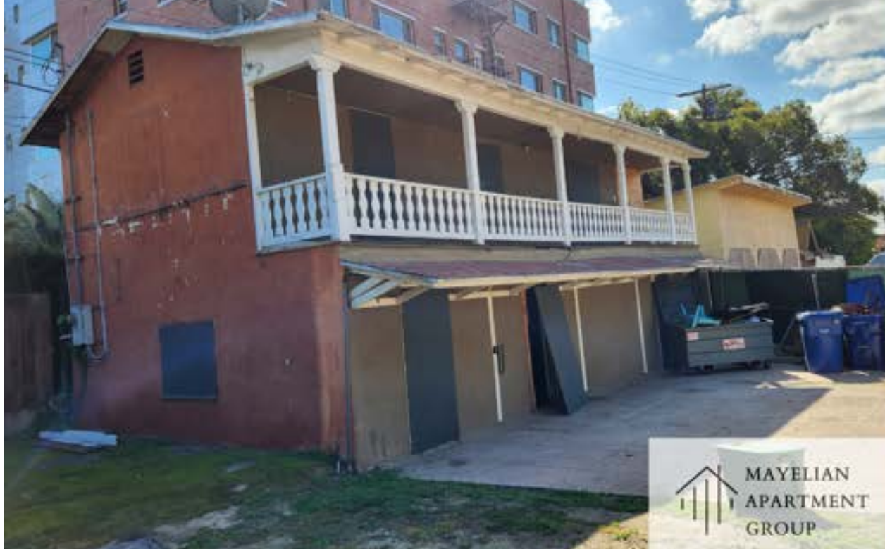
BEFORE (BACK BUILDING)
