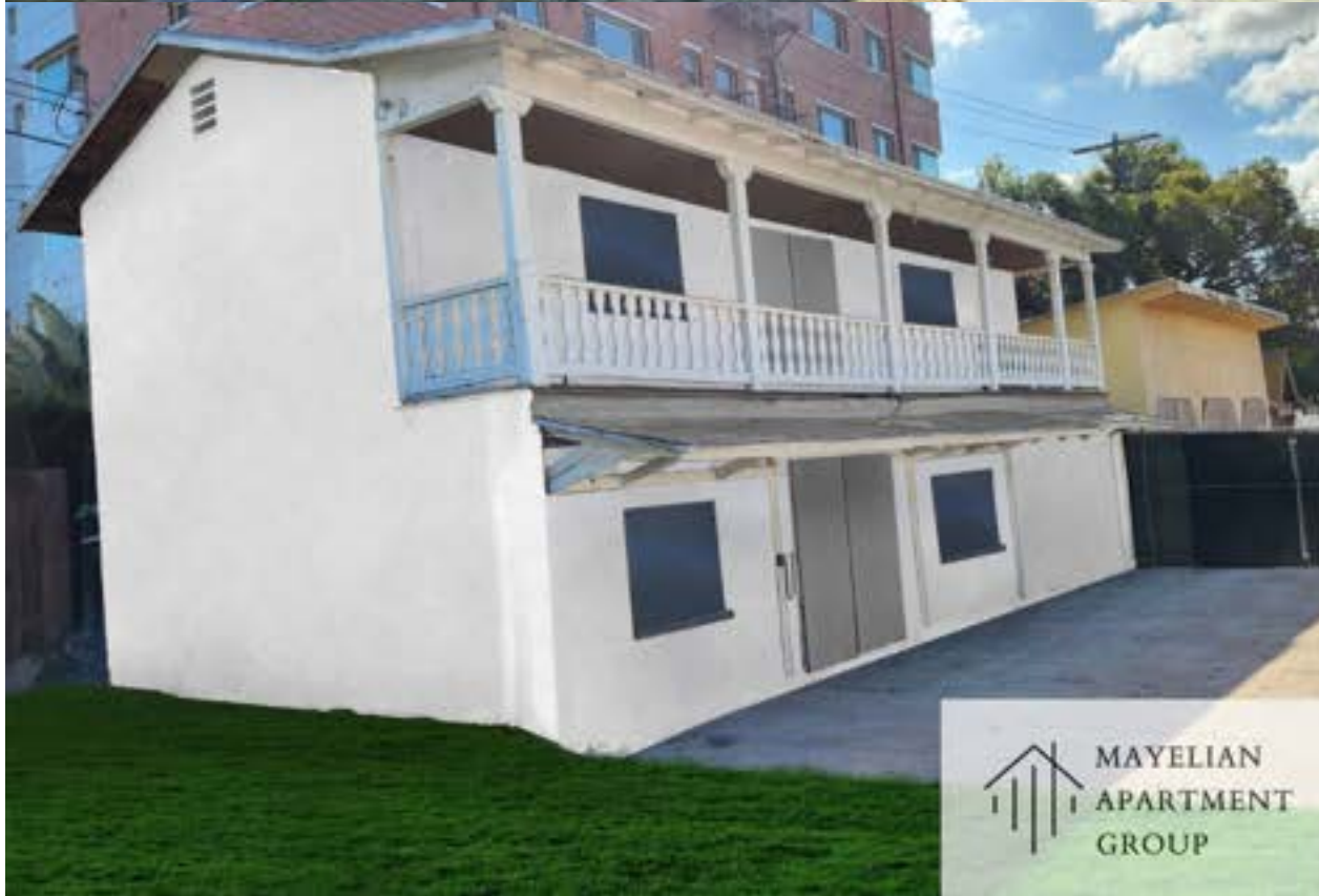
AFTER (BACK BUILDING)
